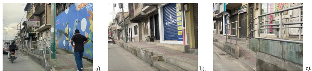
FIGURE 4. EXAMPLE OF IDENTIFIED ISSUES.
